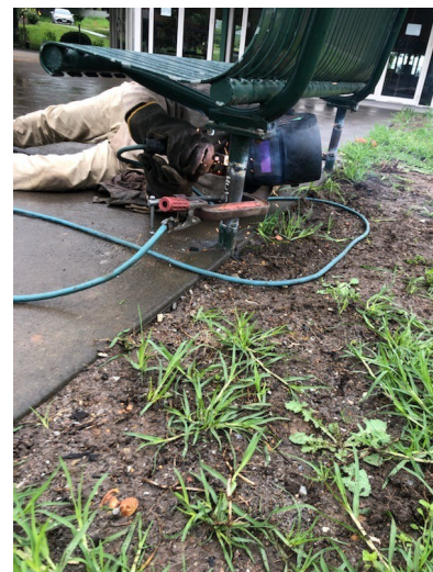
Andrew lifting the height of the seating out the front of the Church.
